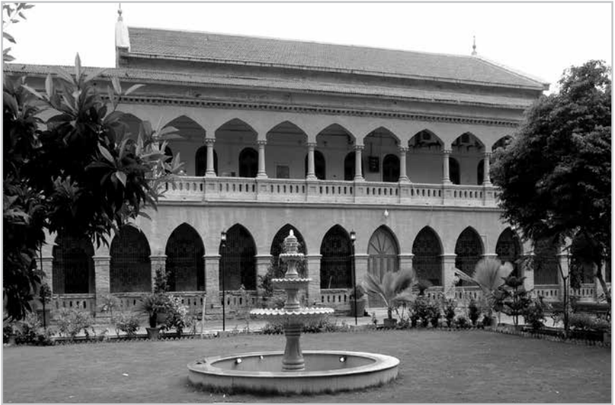
Main Building of Sindh Madressatul Islam University, Karachi.
